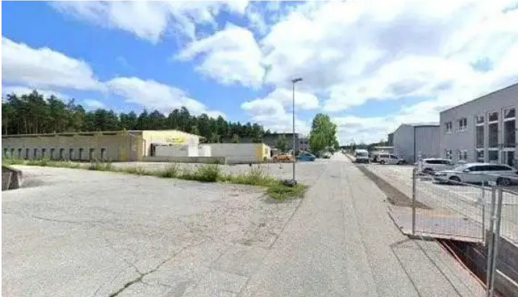
Esc energy systems company alle
