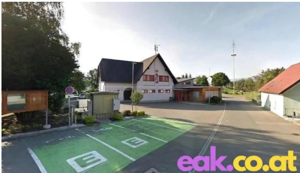
Energie steiermark charging station kobenz
