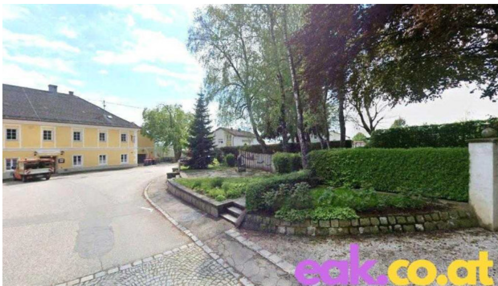
Energie ag charging station bachmanning
