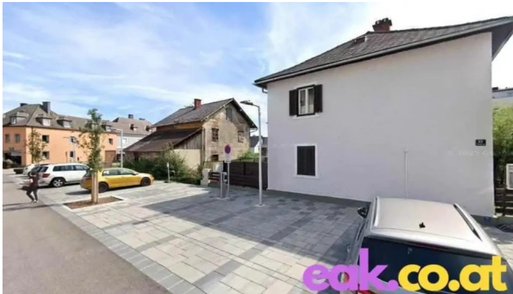
Energie ag charging station attnang puchheim
