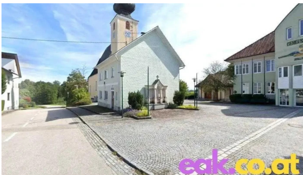
Energie ag charging station 45
